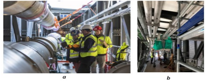
Figure B.1.11: Installed Cryolines at ITER site.
