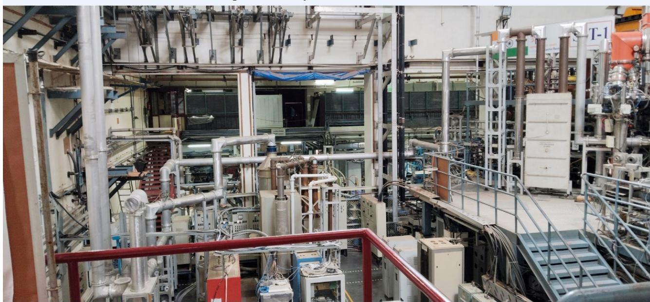
Figure A.1.34: Newly installed Aluminium transmission line and matching network at SST-1.
