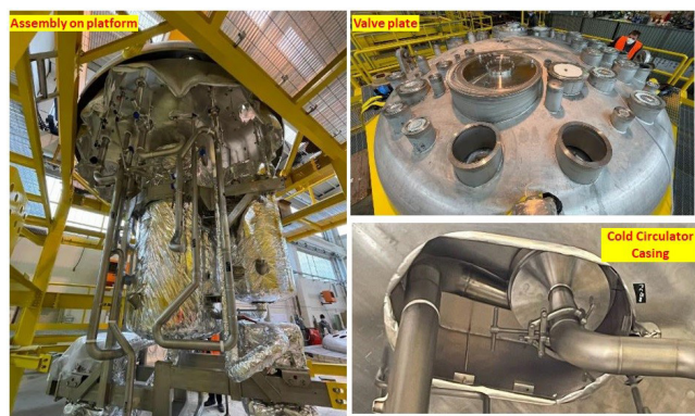
Figure B.1.10: ACB assembly under progress.
