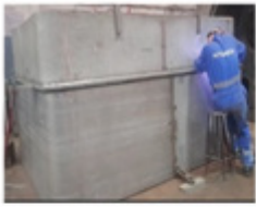
Sub-Assembly A1 Welding completed
