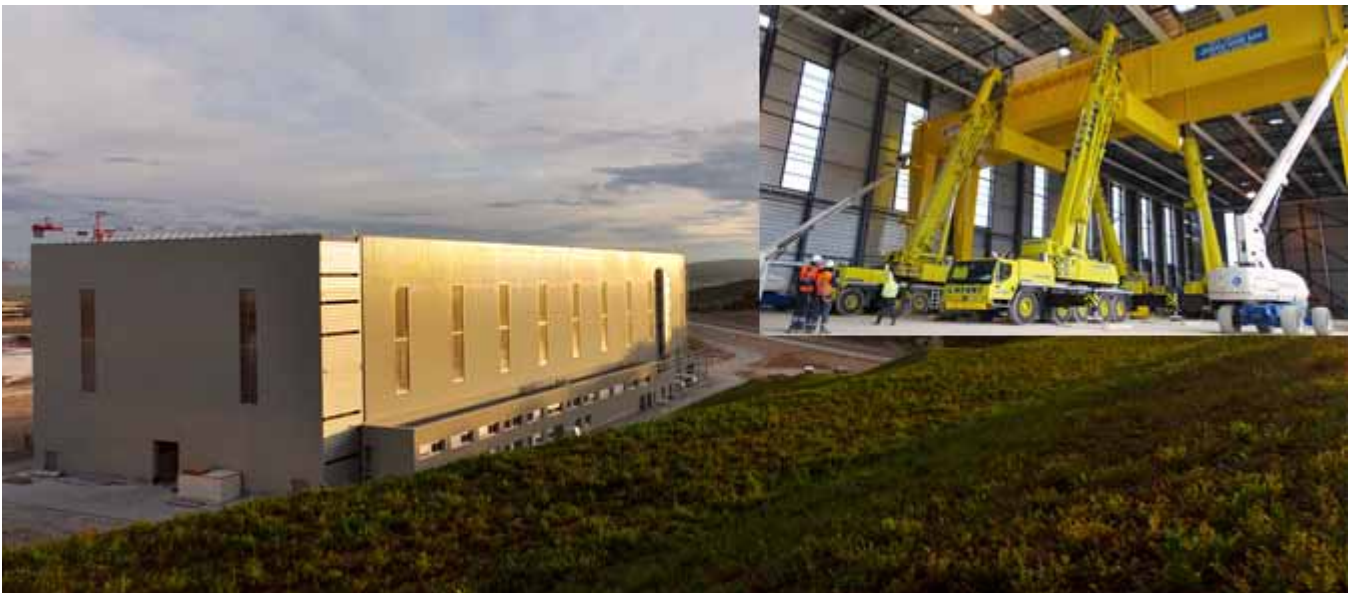
Figure B.2.2 Cryostat Workshop at ITER site, Cadarache, France and crane installed inside
