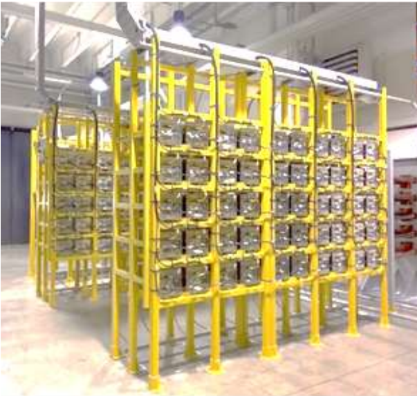
7.2 MW, 96kV HVPS operational at SPIDER facility, ITALY
