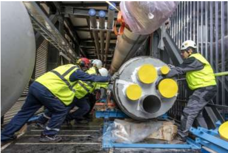
Installation of the seismic decoupling spool being carried out at ITER site
