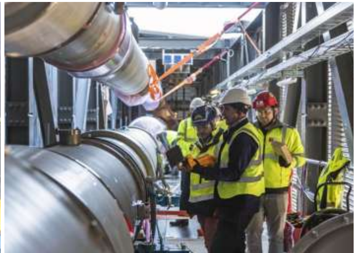
Installation of the seismic decoupling spool being carried out at ITER site
